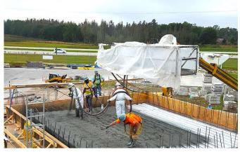
To demonstrate the effectiveness of the Nebraskadeveloped shielding concrete, ABC Group recently built and tested a prototype structure at its disaster recovery complex in Lakeland, Florida. The structure exceeds military shielding requirements. Credit: ABC Group LLC
