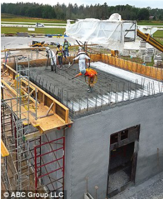
The EMP-shielding concrete could be applied in a spray-on technique that would allow for cost-effective retrofitting
