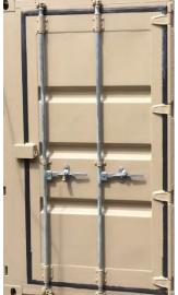
Figure 31. Sample door with gaskets protecting against EMP threats
